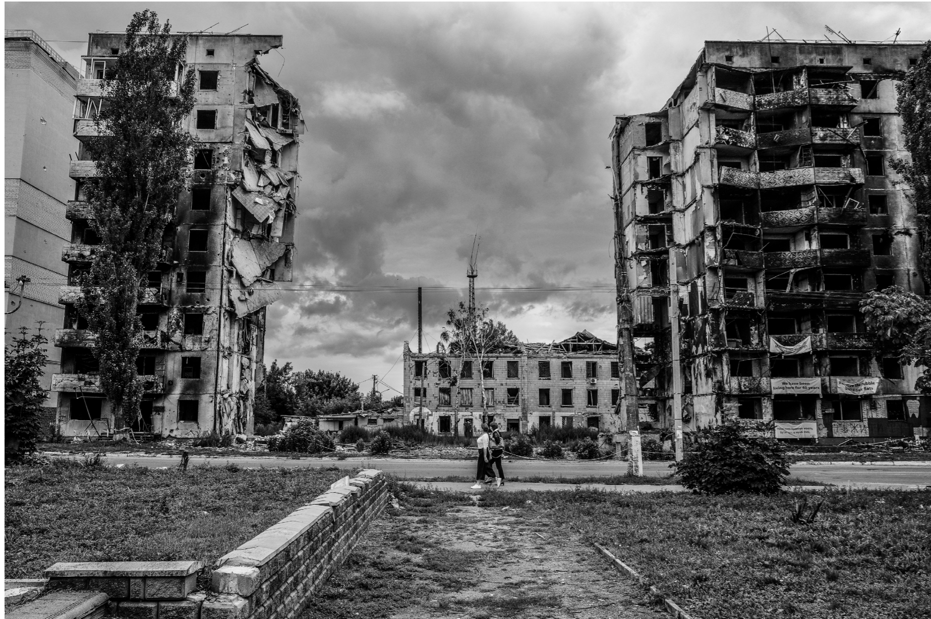
↑ Indiscriminate Russian tank, artillery and rocket attacks have caused massive destruction across many towns and cities. Borodyanka, August 2022.
