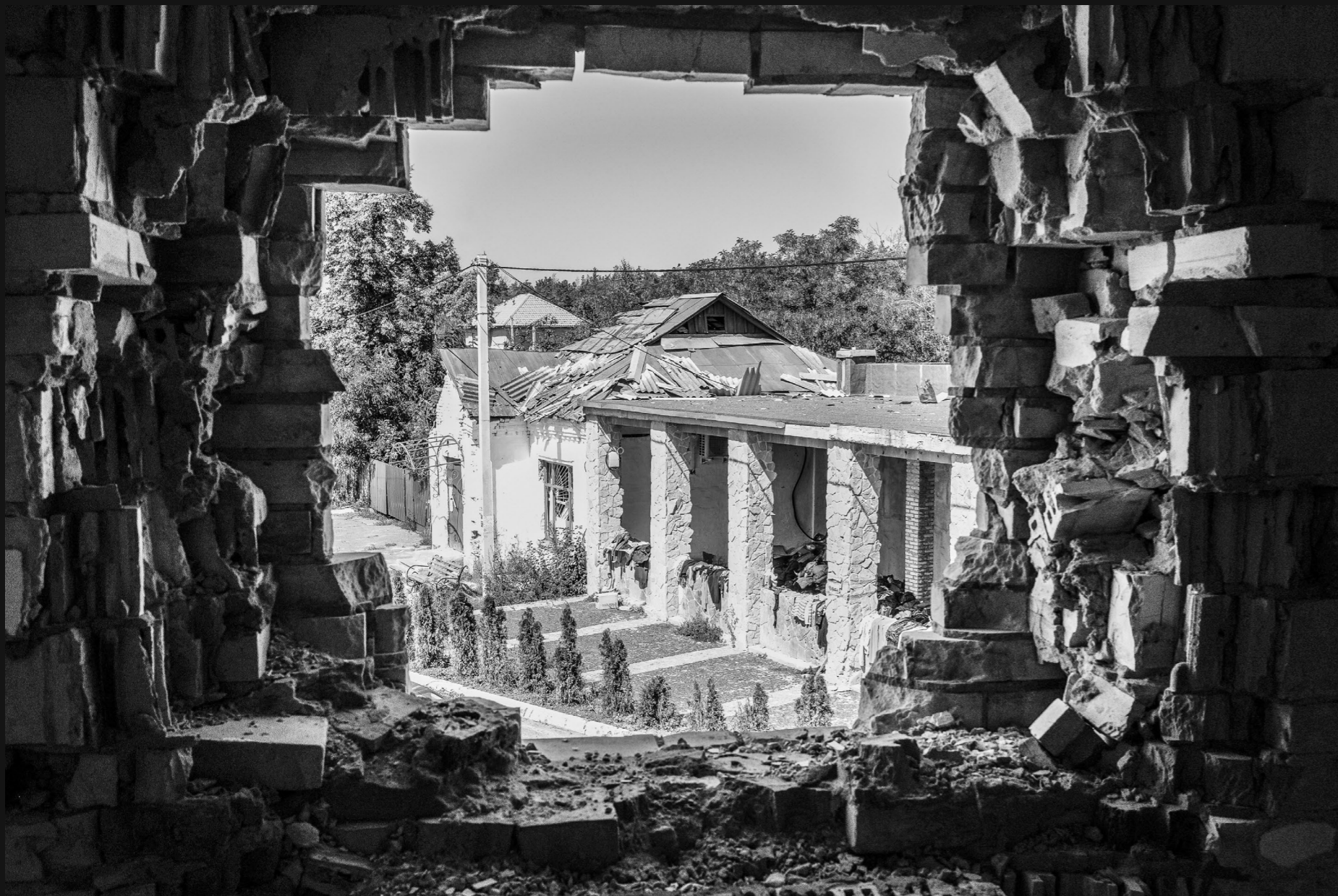
↑ View through shell hole in a village where 85 percent of houses were destroyed or damaged. Moschun, August 2022.
